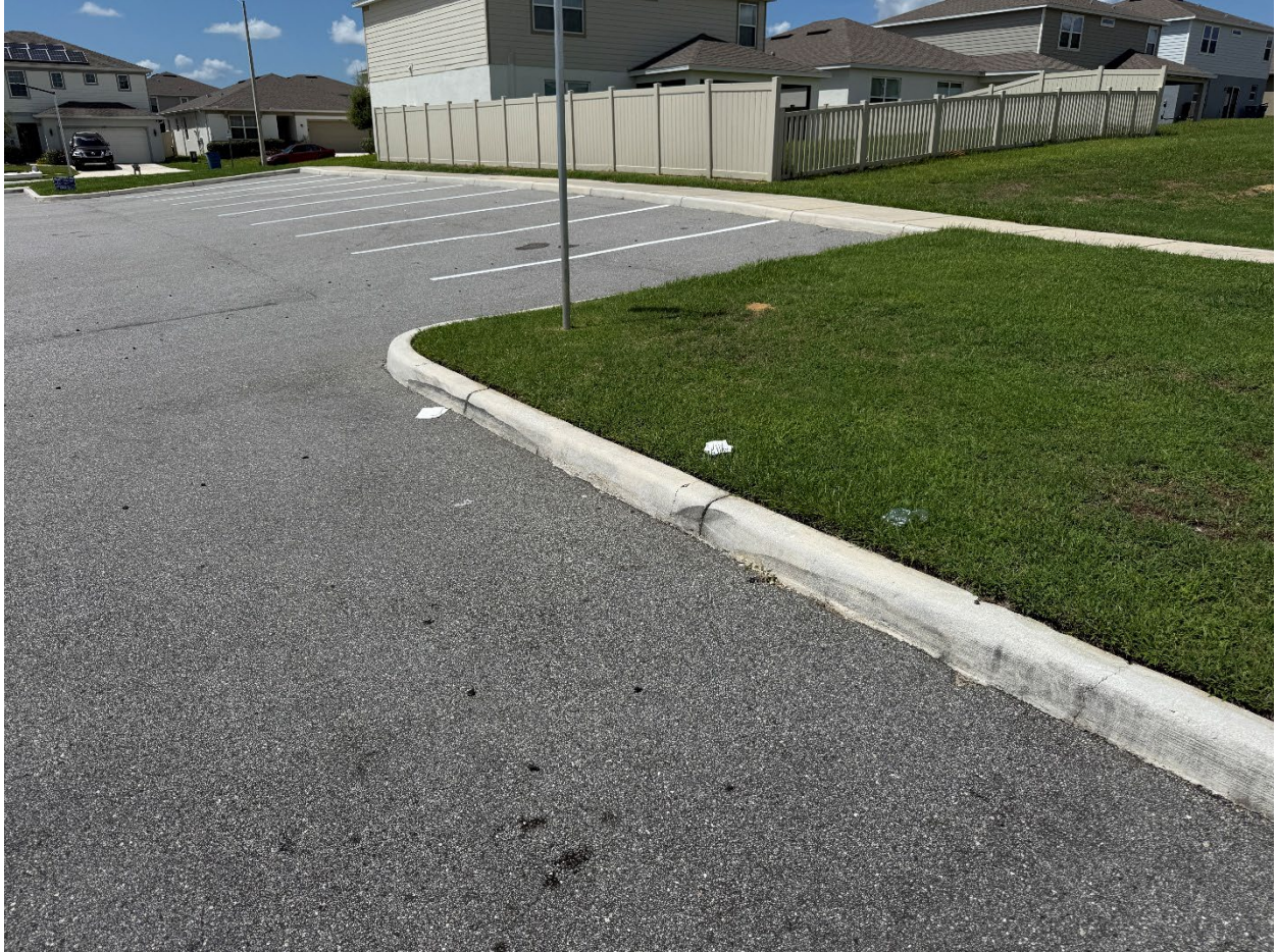
Trash and debris outside pool and playground area
